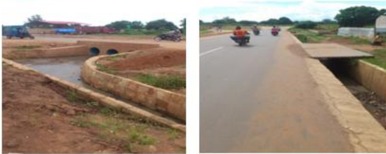
Fig7: Drainage ditches where ravines were located.
